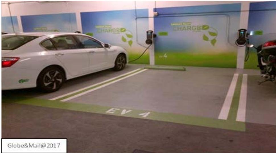
This is a photograph of what *electric vehicle supply equipment* might look like when installed in several parking spaces in a garage
